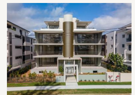
IVY KINGSCLIFF LINK BUILD CONSTRUCTION
