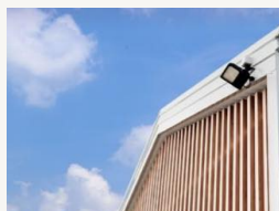
EDEN EARLY LEARNING · APRIL 2023 GREENBANK NORTH CONSTRUCTION
