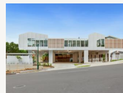
GUARDIAN CHILDCARE · 2024 EATONS HILL NORTH CONSTRUCTION
